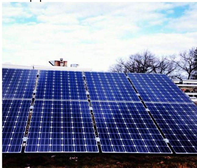
Completed installation showing gaps between panels
