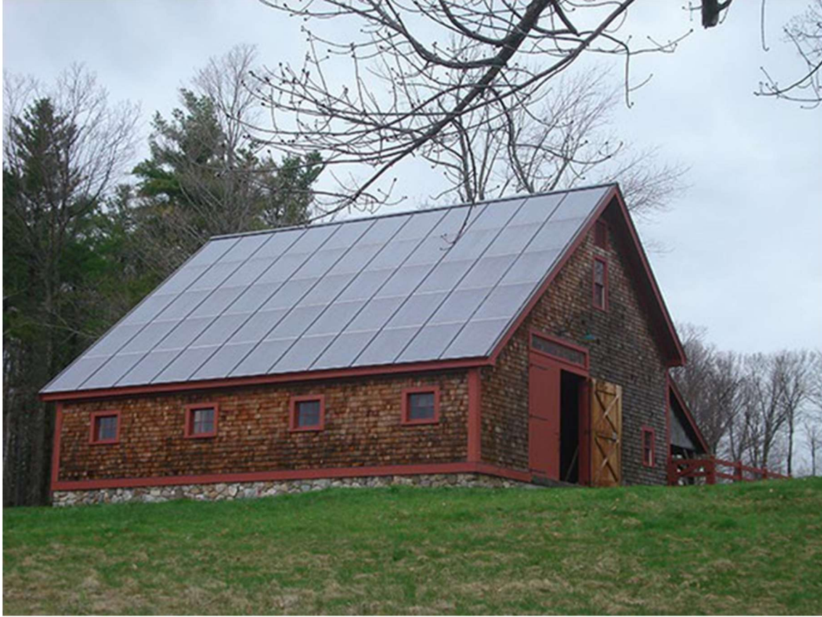
Great Hill Farm barn in Tamworth
