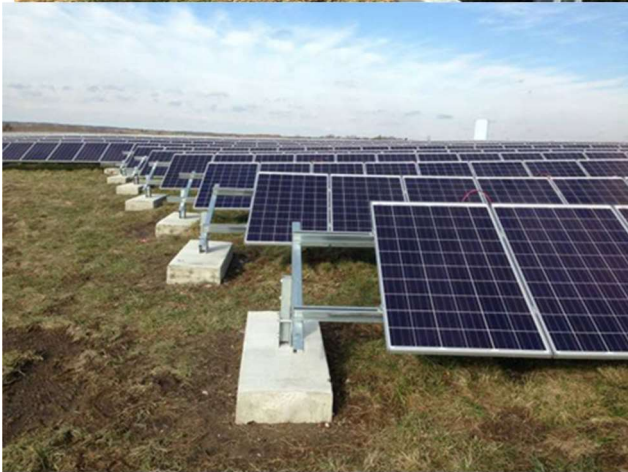
Ballasted system, showing the distance between rows and the ballast blocks.
