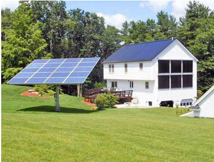
Tracker Mounted Residential System: Courtesy Revision Energy
