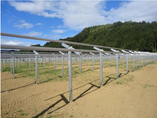
Racking equipment – before panel installation.
