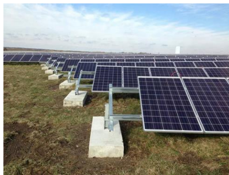
Ballasted system, showing the distance between rows and the ballast blocks.
