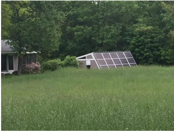
Residential Ground mounted system.
